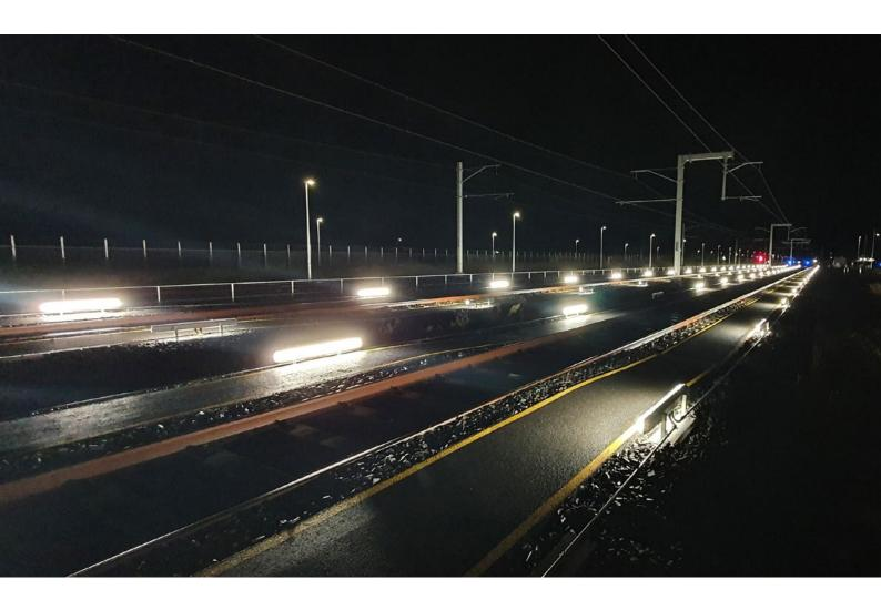
614x fittings installed at the Pakenham Stabling yard 2ft above ground level on the sides of the tracks.
